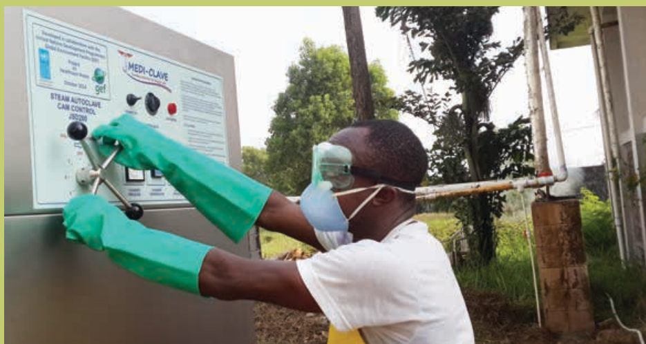
OPERATOR JEFFREY AT JFK MEMORIAL HOSPITAL IN MONROVIA, LIBERIA, TESTING THE NEWLY INSTALLED STATE-OF-THE-ART AUTOCLAVE WHICH WILL BE USED FOR ENVIRONMENTALLY SAFER TREATMENT OF EBOLA HEALTHCARE WASTE. THIS IS DISCUSSED IN MORE DETAIL IN CASE STUDY #10. PHOTO BY BABACAR NDOYE.
