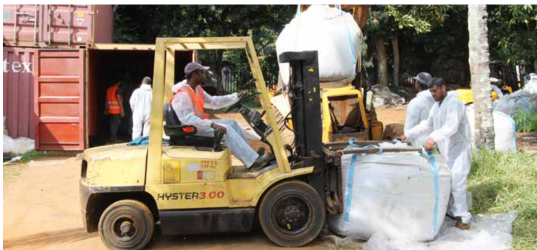
PACKAGED DDT CONTAMINATED SOIL IS LOADED INTO SHIPMENT CONTAINERS AT PAMPLEMOUSSES, MAURITIUS. PHOTO BY HILDA VAN DER VEEN.
