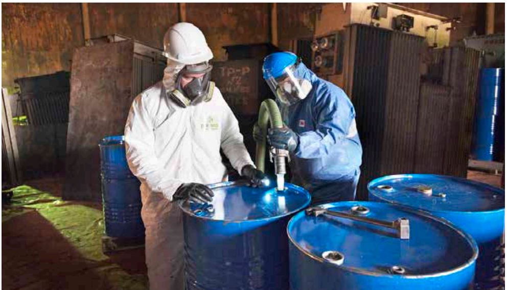
DRAINING OF PCB OIL FROM TRANSFORMERS AT ARCELORMITTAL TEMIRTAU IN KAZAKHSTAN. PHOTO BY POLYECO.
